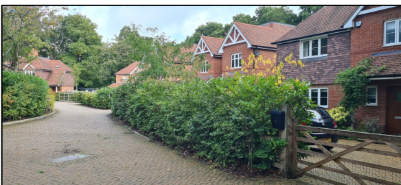
Laurel Bank (top and middle photographs) on Harts Lane and Sandham Gardens on Pound Lane (bottom right photograph). Cul de sac style developments which have responded well in their use of a variety in architectural detailing, style and materials and maintaining the intimate and enclosed character of the area in landscaping schemes.
