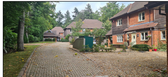
Cul de sac style development at Stembridge Close a good example of the use of a variety in architectural detailing, style and materials and maintaining the intimate and enclosed character of the area in landscaping scheme. The use of kerbing on both sides of the road introduces an urbanising influence.
