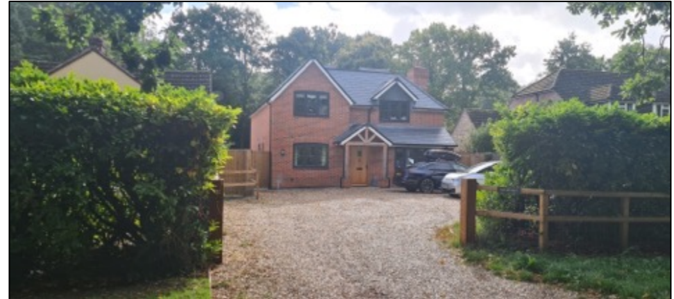
New development on Pound Lane. Use of chimney stack adds interest to roofscape and entrance porch adds interest to street scene. Use of black roof tiles out of character. Strong hedgerow structure and informal road treatment maintained.
