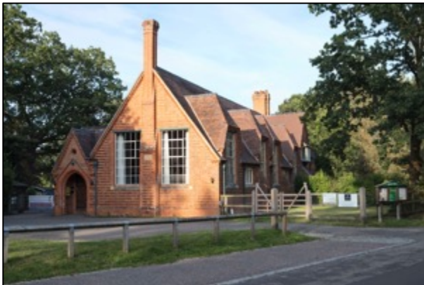
Grade II listed Portal Hall (Parish Room and House)
