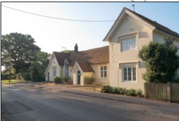
Locally listed Burghclere Primary School
